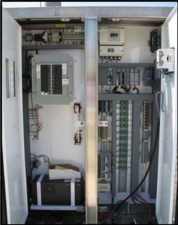
San Sevaine Turnout control panel
