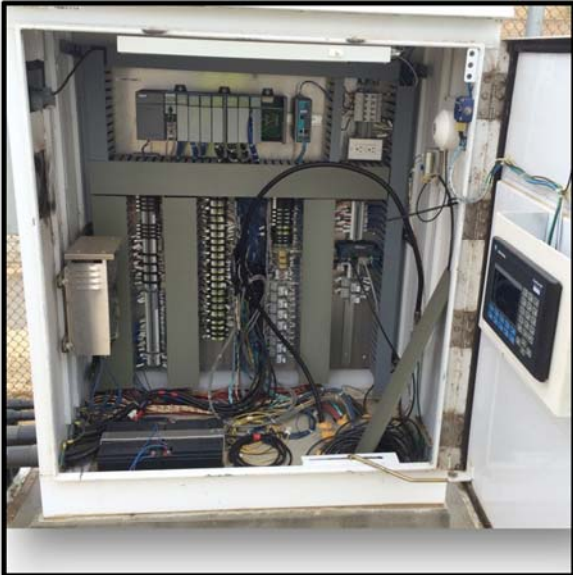
Turner Basin control panel
